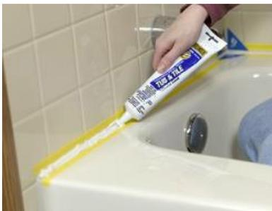
Maintaining these areas is easier and less expensive than making the costly repairs that are necessitated by water damage. On an annual basis you should inspect the areas if the existing caulk is discolored or has mildew on the surface, it can be cleaned by using commercially available cleaners or general household materials such as bleach, baking soda, distilled vinegar, or peroxide. If the existing caulking is dry, loose, damaged, missing, or stained, it should be removed and replaced.
