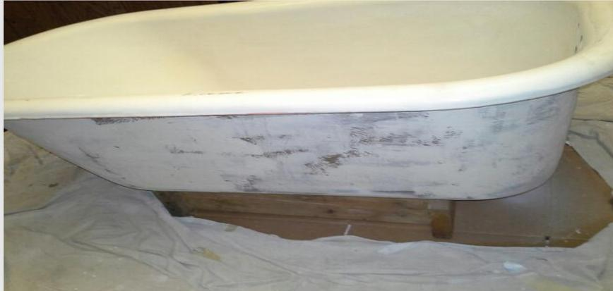
**Using polyester filler we go around your tub, filling in holes and low spots.**
