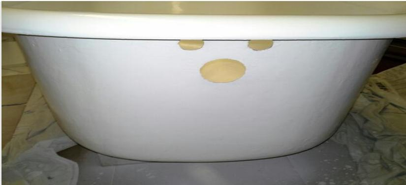
**After sanding the high build primer the exterior gets polyester bonding primer and multiple coats of polyester protective top coat.**
