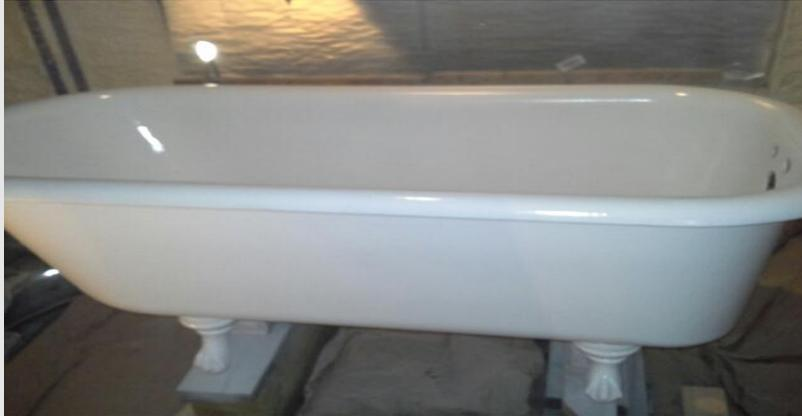
**With the outside completed and masked off. The clawfoot is flipped over and the same steps are repeated for the inside of the clawfoot tub.**
