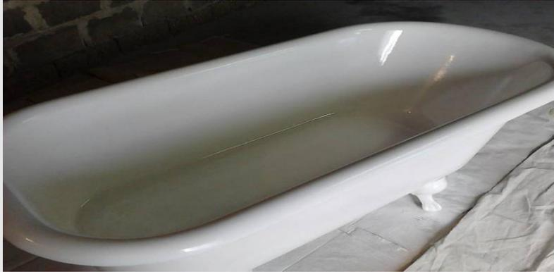
**Applying multiple coats of high build chemically hardened primer.**
