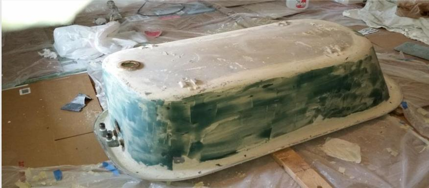
**Sanding the filler levels out the casting defects.**
